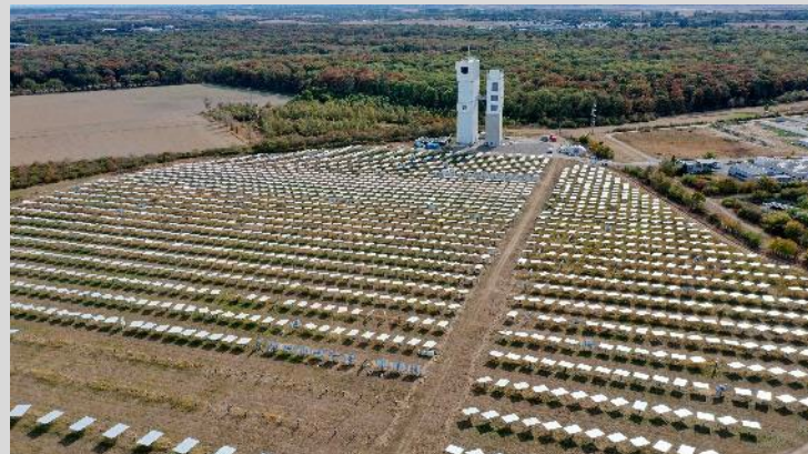
DLR Solar Towers
