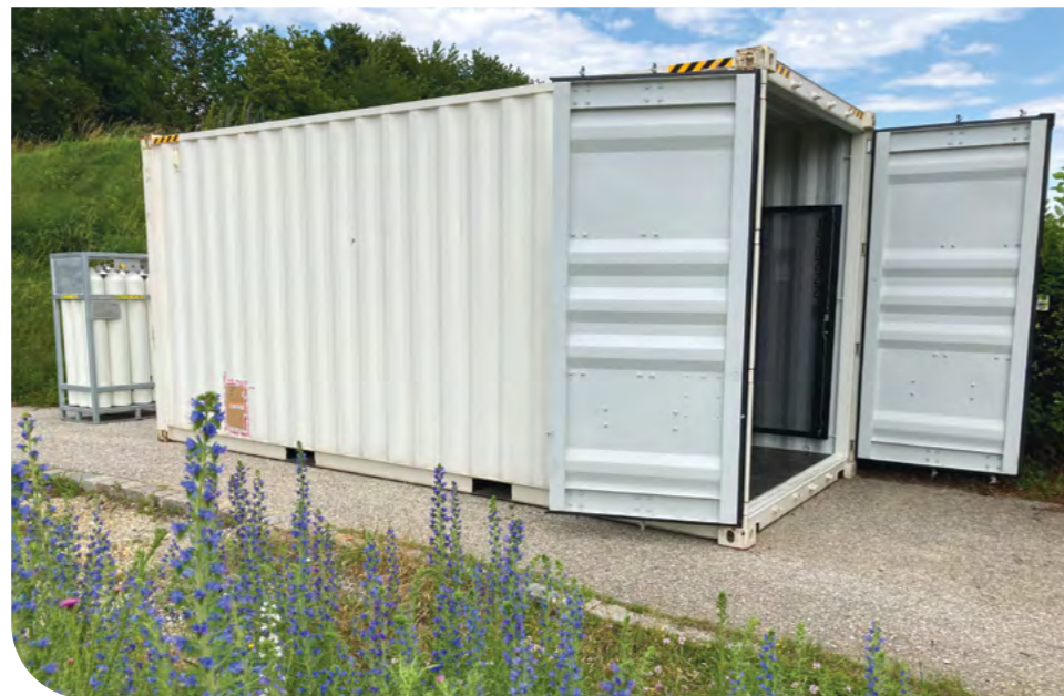
Figure 4: P2P H 2 -Demonstrator overall set-up with 20-ft container and hydrogen gas storage.
